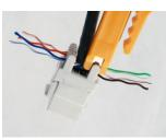
Use the insertion tool (partnr. 39931.1) to punch down the wires into the LSA-contacts
